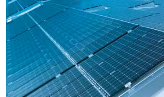
Photovoltaic modules on the roof generate sustainable energy for production facilities and office buildings.
