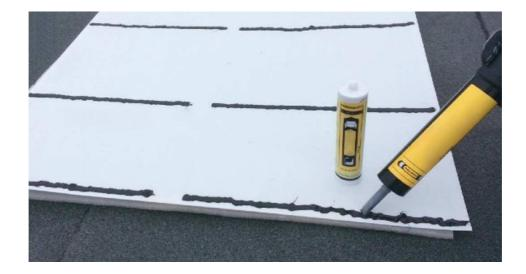
The adhesive lines can be as close to each other as required (the number of lines depends on the strength your chosen adhesive), but a minimum gap of at least 70 mm between lines is recommended. In general, for most plastic / fibreglass / metal surfaces
